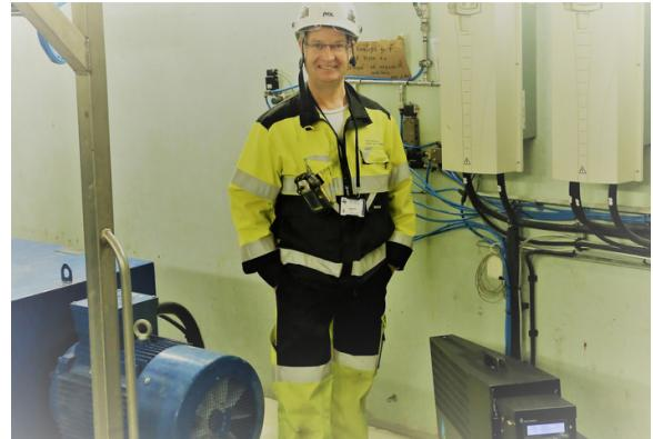
Previously, this station relied on direct-acting electric heating (with an installed power of 4650W) and ventilation, yet it still faced moisture issues. The pump station, measuring 40m<sup>2</sup>, houses three pumps, each capable of pumping 160L of wastewater per second.
