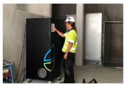
ventilation pipes. This means that all energy stays inside the building. The condensed water is easily led to the nearest drain and as the dehumidifiers are mobile it has been possible to reposition one or two of the machines inside the building to address temporary local humidity load.
